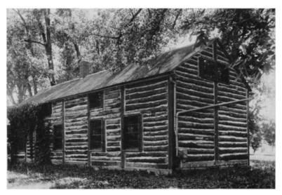
Fig 6 Pièce sur pièce Construction (Source: Dr. Fred Kniffen and Henry Glassie, (Article: SocietyBuilding in Wood in the Eastern United States: A Time-Place Perspective, Geographical Review, Vol. 56, No. 1 Jan., 1966, Published by: American Geographical Society), Accessed from Jstor archive, [http://www.jstor.org/stable/212734])
