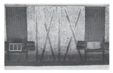
Fig. 4 Brique Entre Poteux Construction (Source: Dr. Fred Kniffen and Henry Glassie, (Article: SocietyBuilding in Wood in the Eastern United States: A Time-Place Perspective, Geographical Review, Vol. 56, No. 1 Jan., 1966, Published by: American Geographical Society), Accessed from Jstor archive, [http://www.jstor.org/stable/212734])
