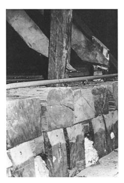
Fig 7 Close studding: external lap tenons support a heavy plate at the Bolduc House, Ste. Genevieve, Missouri, ca. 1785. (Source: Jay D. Edwards, Creole Architecture: A Comparative Analysis of Upper and Lower Louisiana and Saint Domingue in Springer. Accessed from Jstor archive Nov 25,2011: http://www.jstor.org/stable/20853104. )
